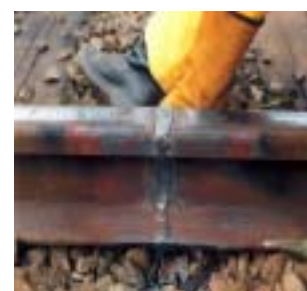
Hardfacing of top layer completed with OK 83-28
