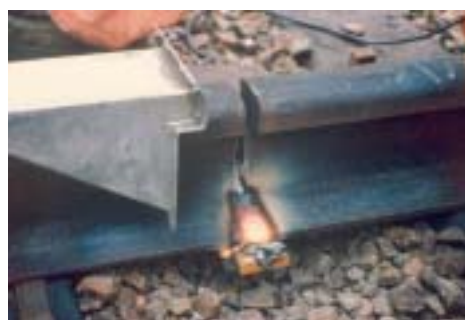
Foot welded with OK 74-78
