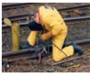
Welding the web of the rail
